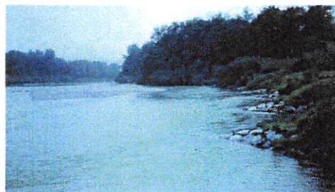
Figure 43: Field installation of stream barbs (USDA, 1996).
